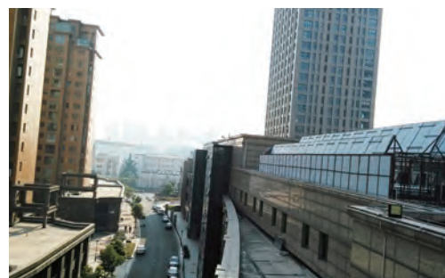
Noise Control of Commercial Building Equipment
