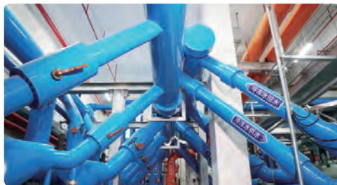
Cold water, hot water, steam pipe outer protection
