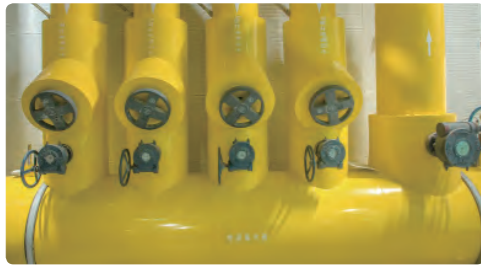
Y-valve outside protection
